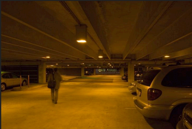
High Pressure Sodium Lighting
