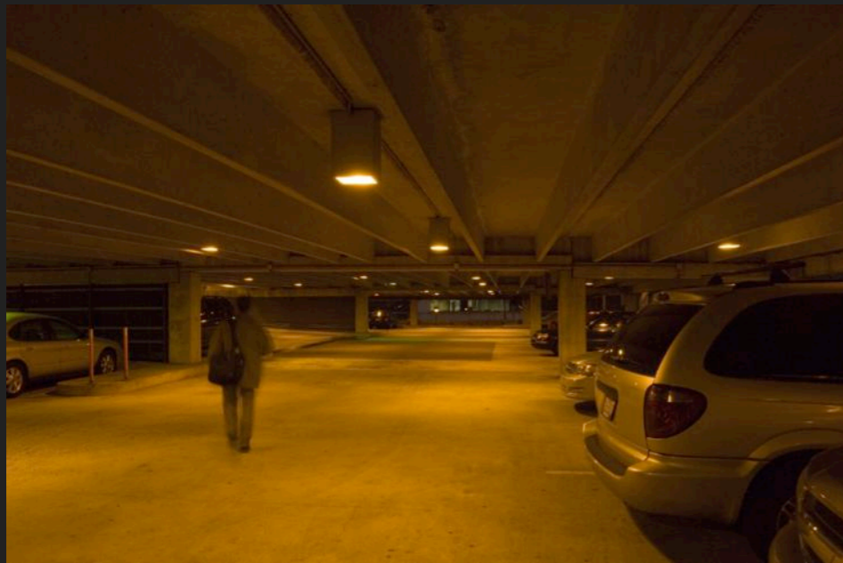
High Pressure Sodium Lighting
